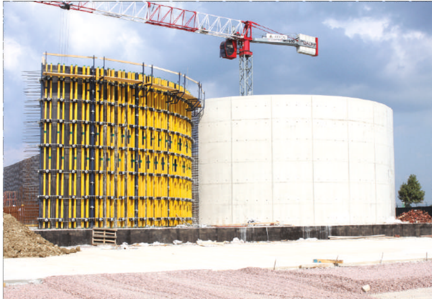
Circular wall formwork wooden beam system's application
