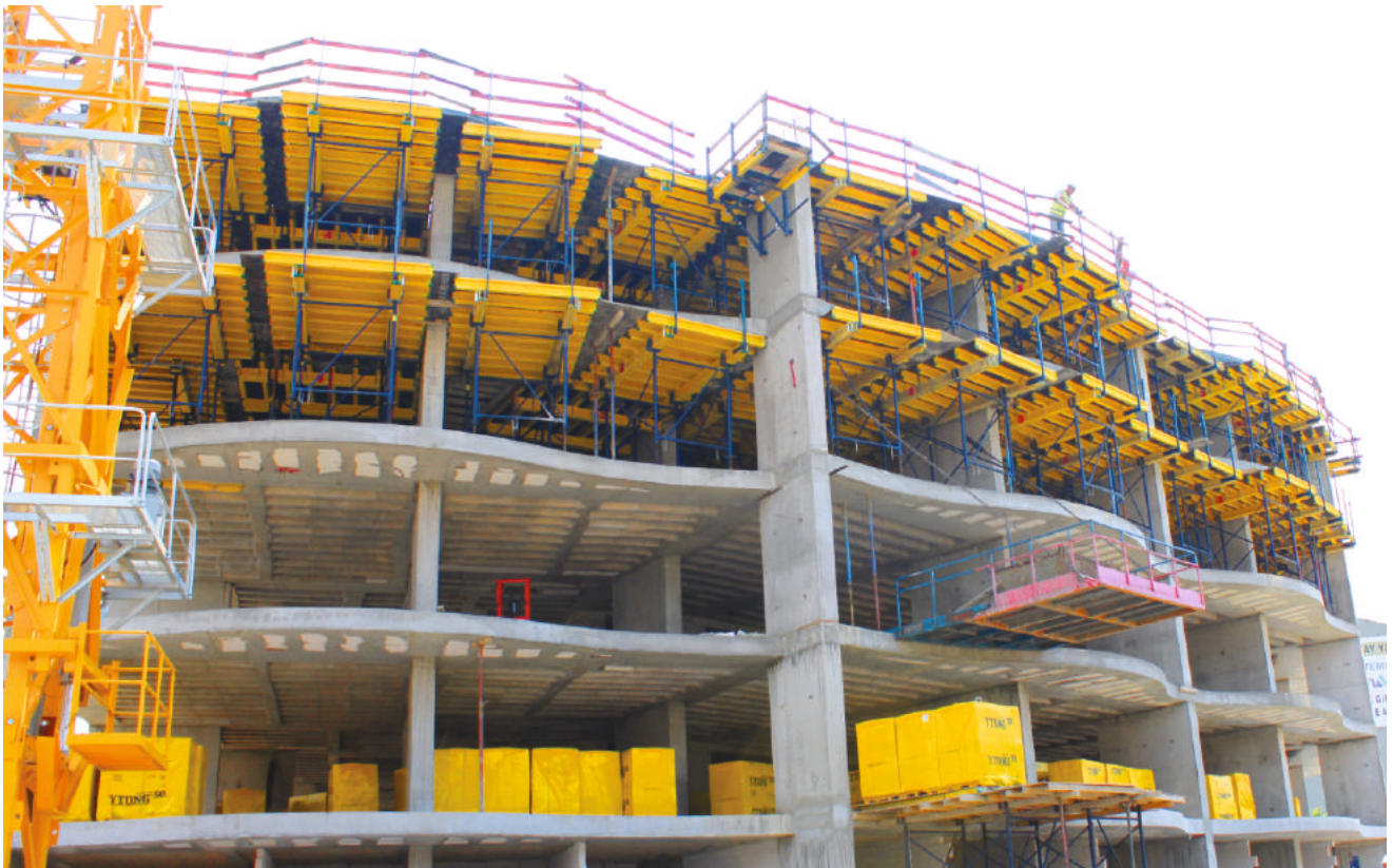
Slabform shoring systems application
