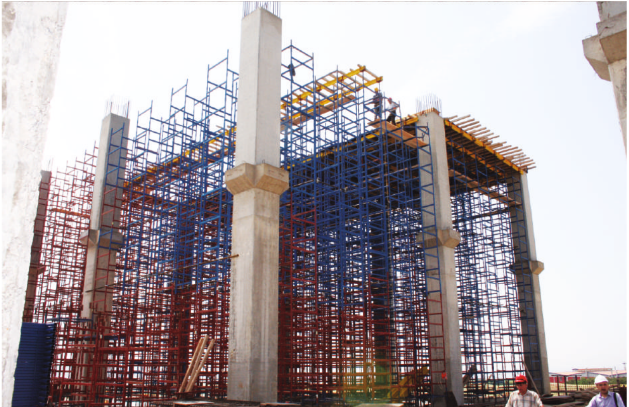
Tower type scaffolding systems application
