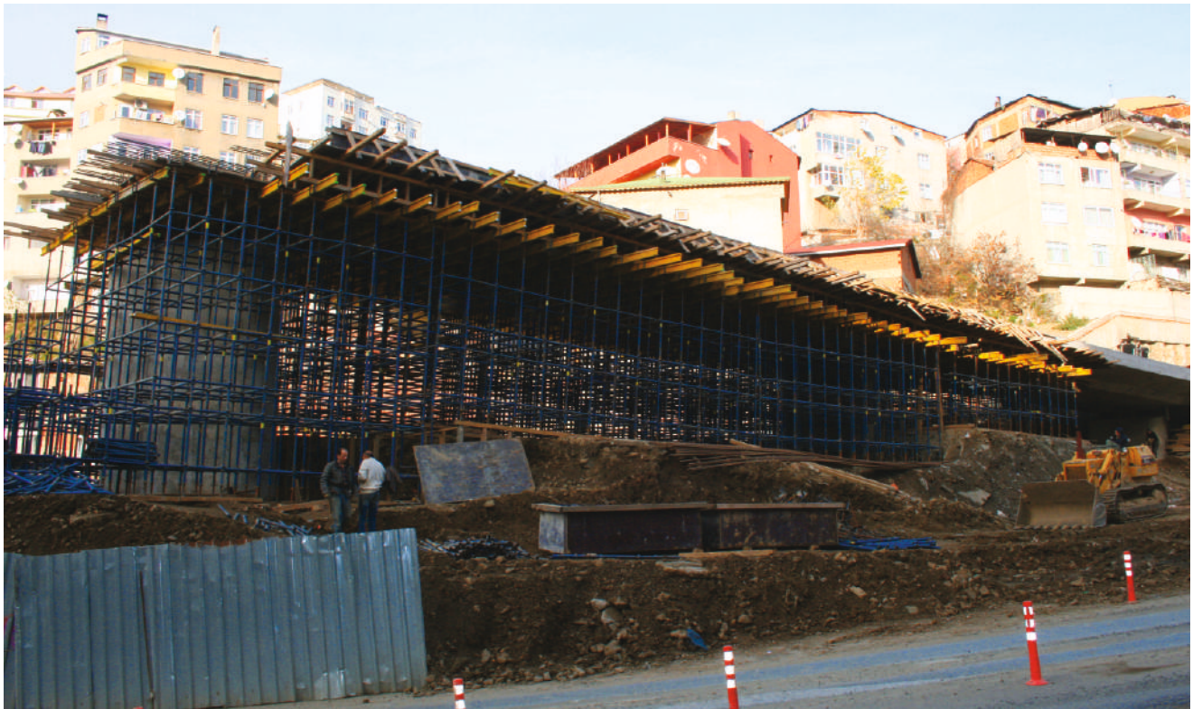
Cup-Lock scaffolding system's application
